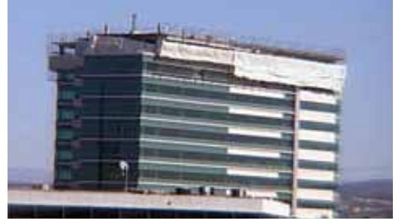
The deconstruction of the top two stories of a San Diego office building located within one mile of Montgomery Fields marked a significant victory for airport protection.
